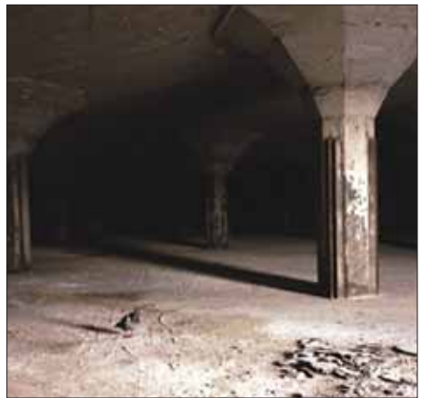
An Interdit Location – Before
