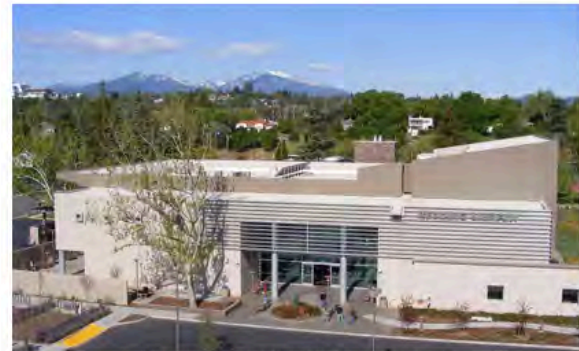
The entrance to the City of Redding public library
