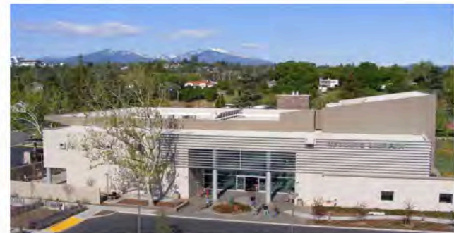
The entrance to the City of Redding public library
